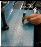
It may be necessary to have some off centre due to chassis mounted equipment. Position and drill.
